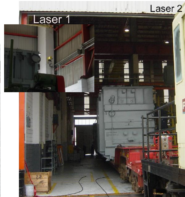
Above is our L-KOPIA/LKO Load Measuring System in Monterrey, Mexico.
